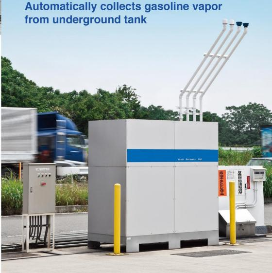
Vapor in the underground tank may cause air pollution or oil loss as vapor is released into the air through the vent pipe.
